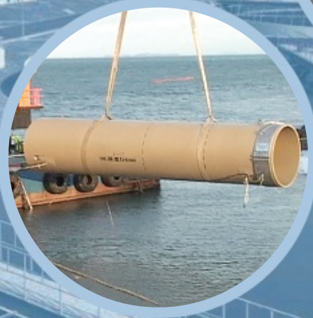
Installation of ocean bed blocks
