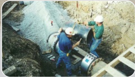
▶ Repair work for pipes replaced underground
