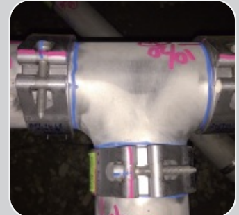
▶ Japan : "T" Repair
