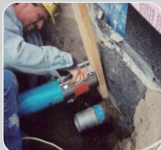
▶ U.S : sewerage repair work
